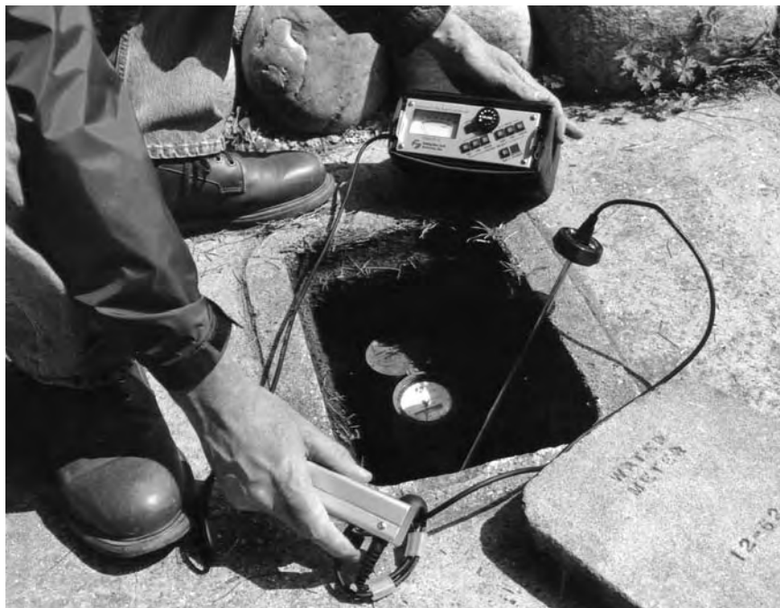
Figure 4-8 Leak Survey at a Meter
